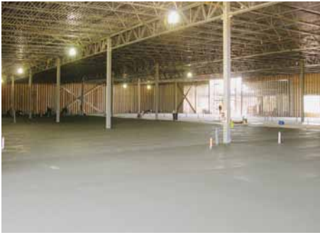
Completing day one of a two-day slab pour.
