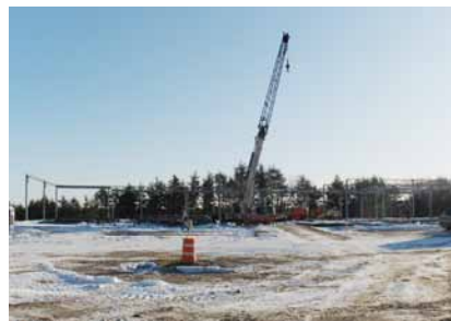
Steel erection at the new Hannaford Supermarket in Gray, Maine.
