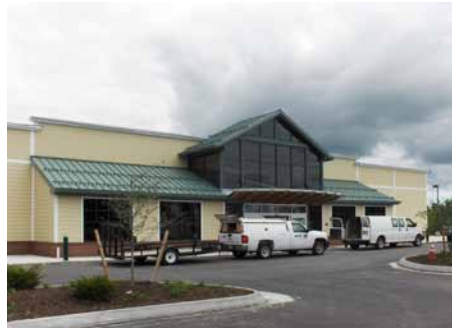
Putting the finishing touches on the new Hannaford Supermarket.
