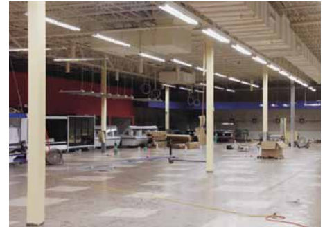
Fit-out of the new interior.
